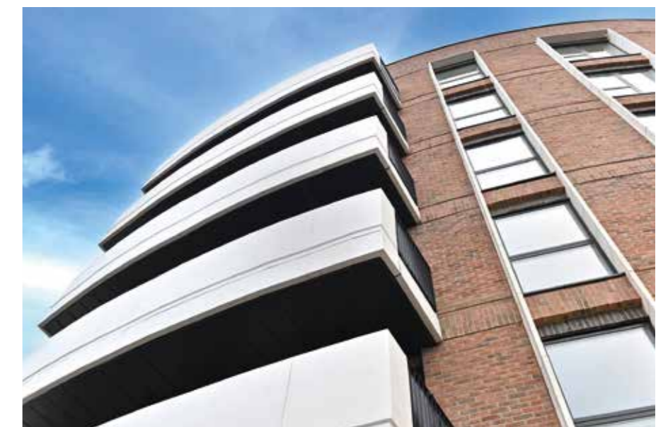
Keith Shaw House, Clapham Park
