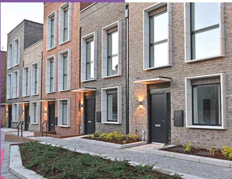
New homes at Clapham Park
