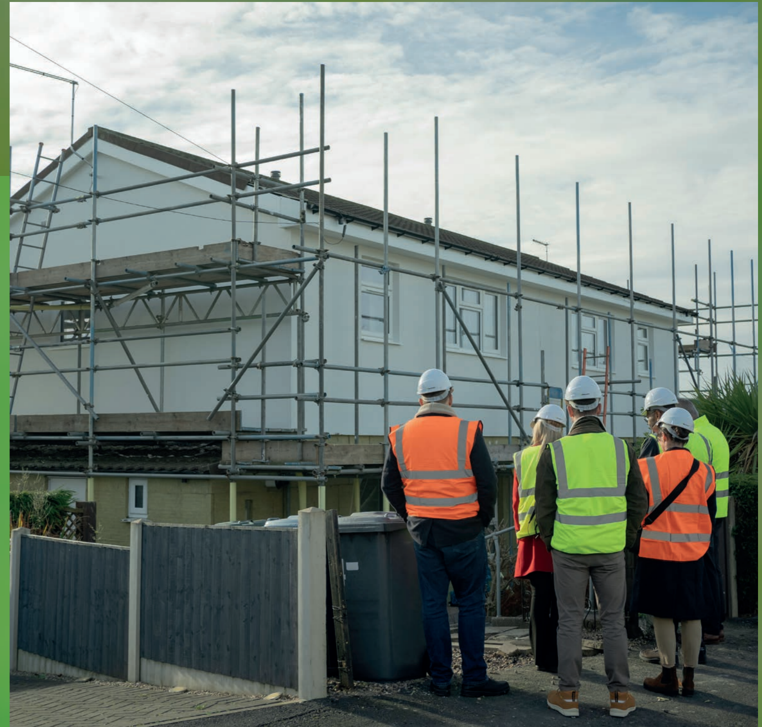
MTVH Decarbonisation Team in East Leake, Nottinghamshire.
